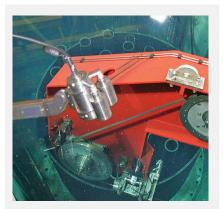
Radiation tolerant cameras used to monitor underwater cutting & dismantling of Reactor components
